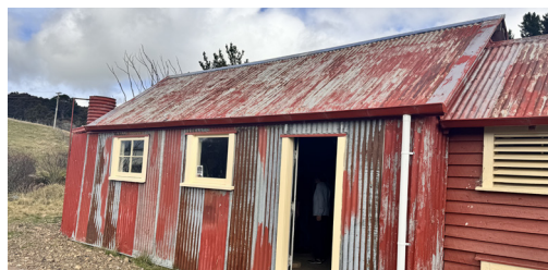
Gentle Annie - Timahanga Station Building
